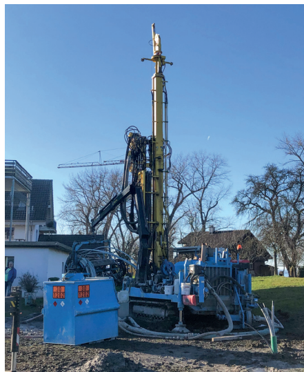
7 GEROtherm®-REX in the drill hole with the drilling rig in the background
