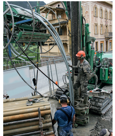
8 The final metres when sinking a total of five double-U 40 mm GEROtherm®-REX probes into the drill hole, each 152 m in length
