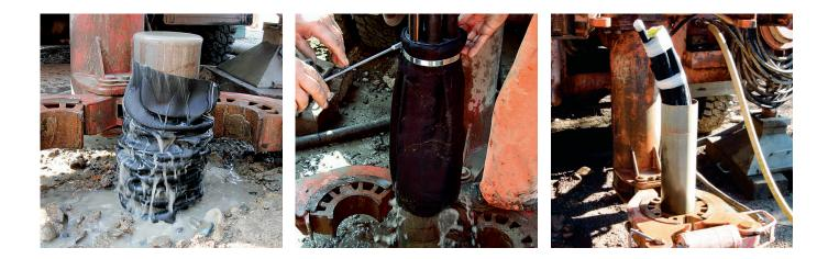
**GEOtight®** (Pat. CH, EU) Patented fabric packer for durable and safe sealing of holes drilled for geothermal probes
