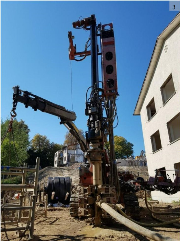
Image 3: Drill rig in use
