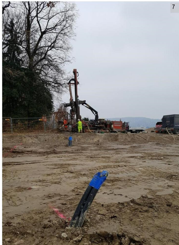
Image 7: Geothermal probes already sunk, backfilled and pressure-tested
