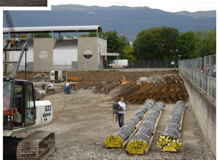
Unloaded, fixed HakaGerodur GEROtherm® geothermal pile probes on the construction site
