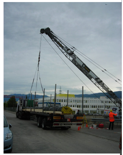
Unloading the GEROthem® geothermal pile probes on the construction site
