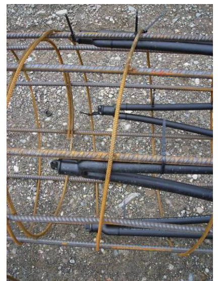
Pile armouring with fixed geothermal probes
