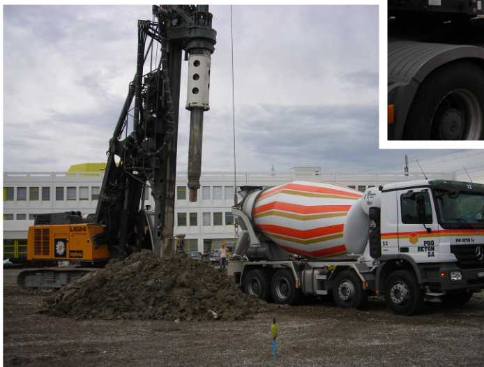
Back-filling the first energy pile
