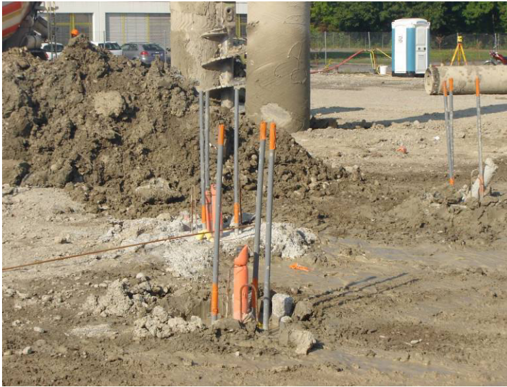
Installed energy piles
