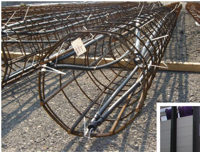
The fixed HakaGerodur GEROtherm® geothermal pile probes
