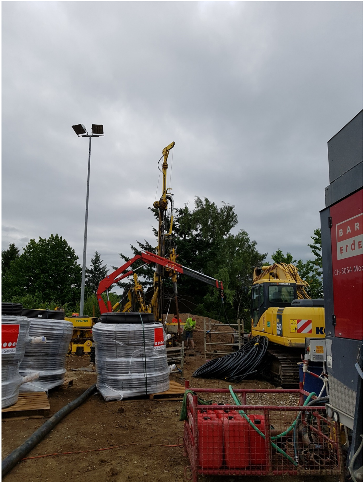
Image legend: Drilling rig with GEROtherm® FLUX probes
