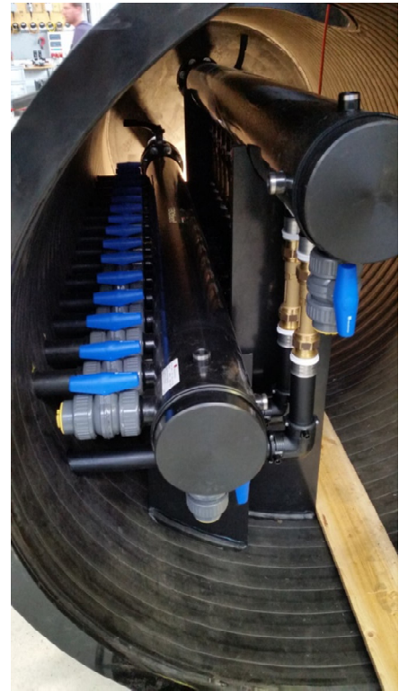
Image legend: Interior view with SAVE 180 collector and distributor
