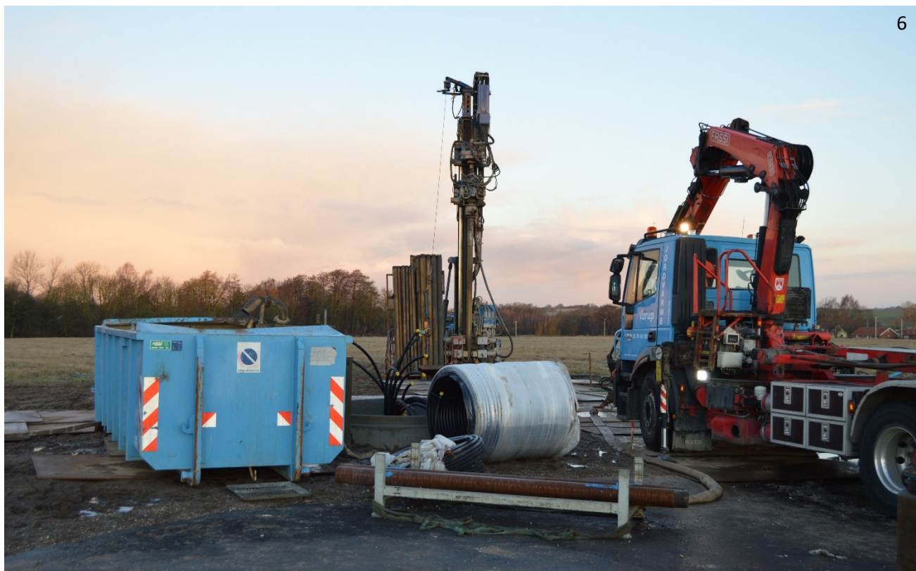
Image 6: Drilling rig Source: www.termonet.dk
