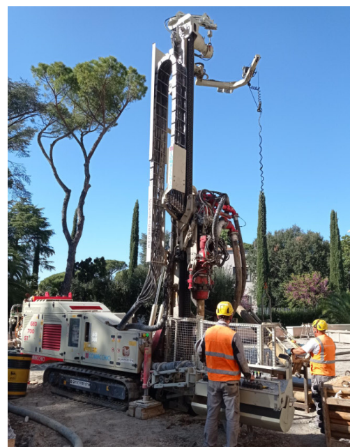
Image 6: The Comacchio GEO 700GT drilling rig Source: Georicerche Srl
