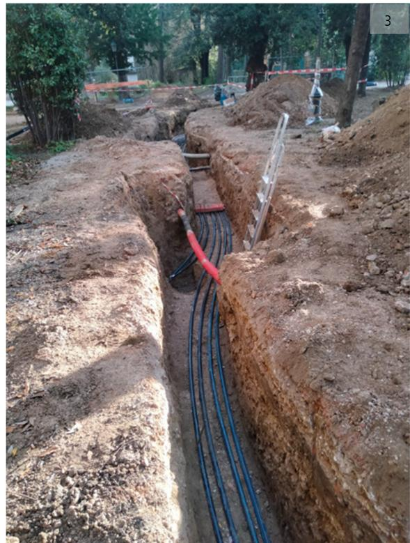
Georicerche Srl also installed the connection pipes and made the connections to six distribution shafts
