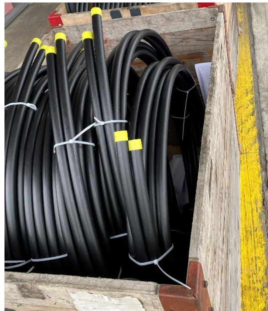
Packing and delivery of the energy piles
