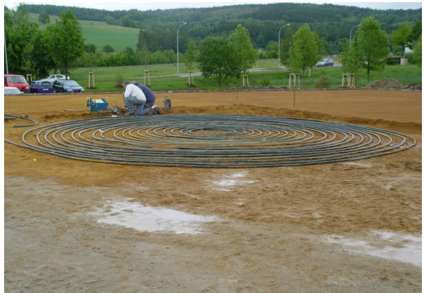
Installation of the heat exchanger
