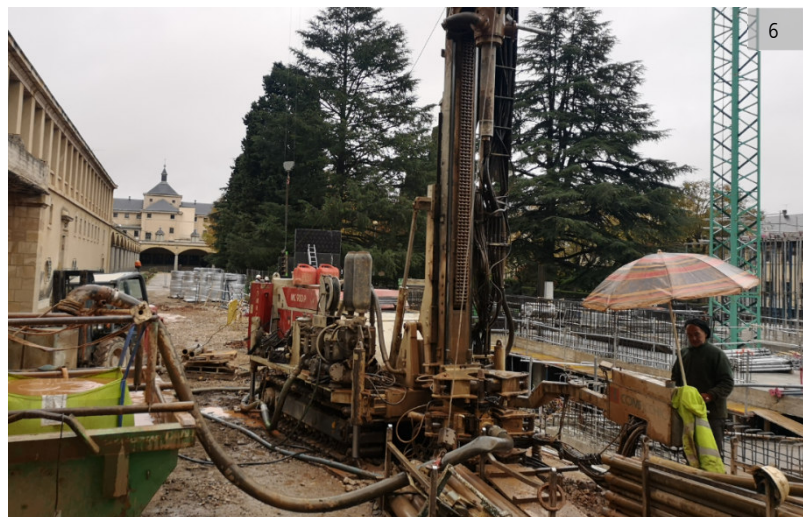
Image 6: Drilling work with Comacchio MC900P Source: HakaGerodur
