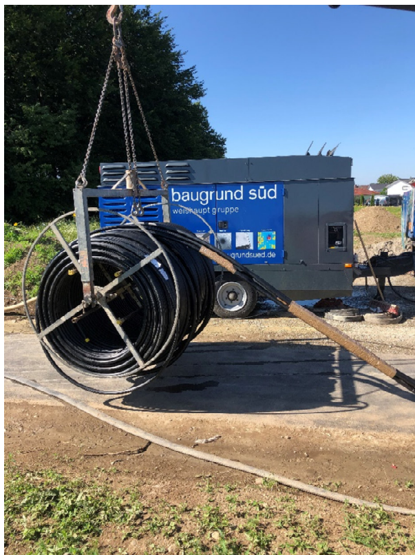
Image 5: GEROtherm® DUPLEX ready for sinking
