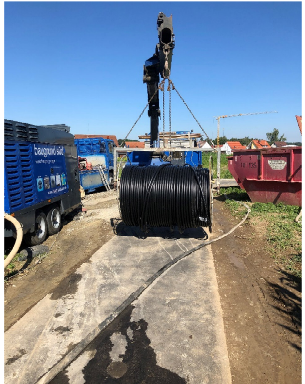
Image 4: GEROtherm® DUPLEX mounted on a reel
