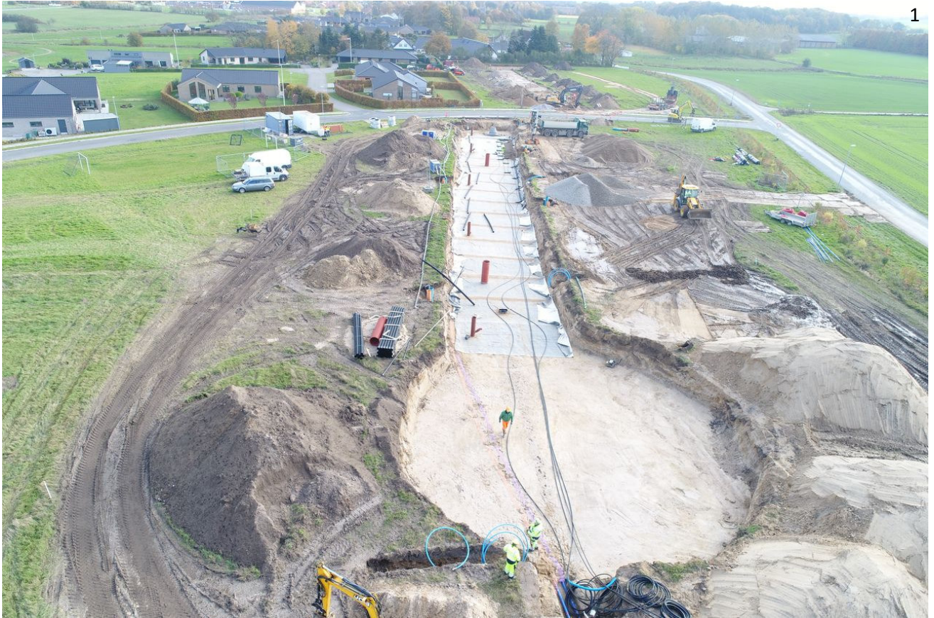
Illustration 1: Chantier Thermoroad Source: www.termonet.dk
